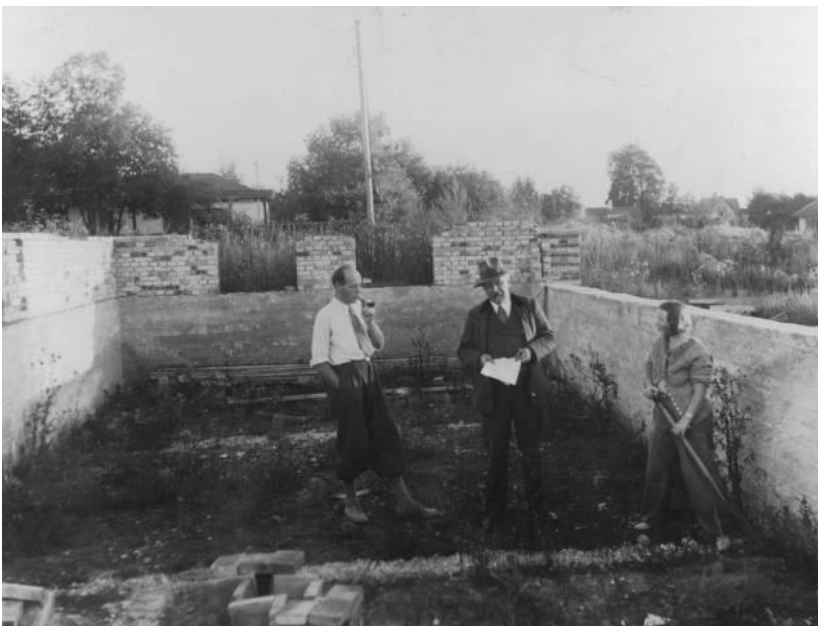
All the Prior brothers were dedicated supporters of TtL, as was architect Knud Brønnum. Here you can see Viggo Prior and his wife, Gertud, together with Brønnum at what was to become their house. The photo is from 1937 and I have found it in the Danish Emigration Archive. Eric Prior donated his entire archive to them.
